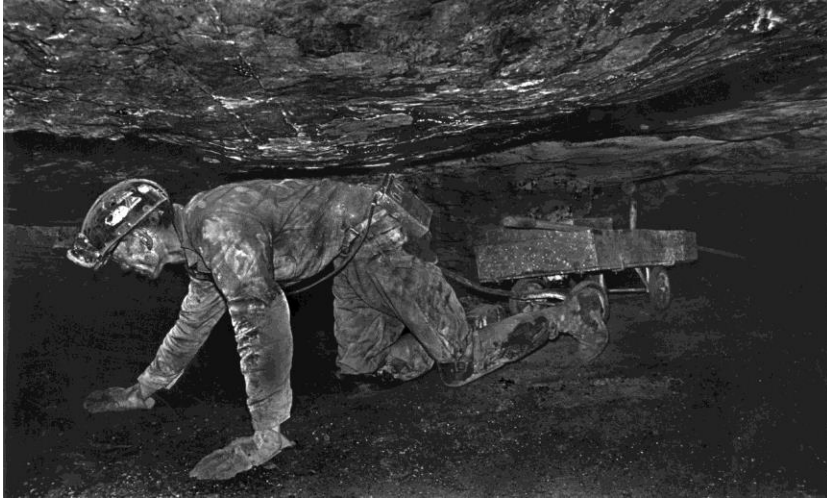
(top) Fireboss performs pre-shift inspection in 30-inch coal seam; and (bottom) using pads on his hands and knees, the shot-firer pulls a wagonload of dynamite to the coal mine face to set the explosives. Logan County, West Virginia, 1976. Photos by Earl Dotter
